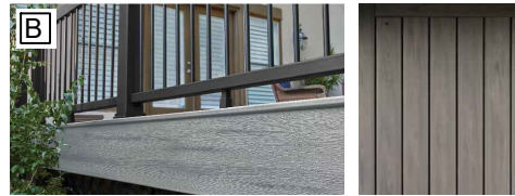
COMPOSITE FASCIA BOARD & SKIRT Style: Trex Fascia Boards & Cladding or similar Color: Clam Shell
