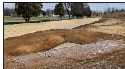
Photo Credit: DNR. Active construction site.
