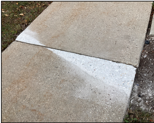
Sample Repair Photo: Defect 23 repaired on 10-22-2024 on Freistadt adjacent to Walgreens at 2:26 PM.
