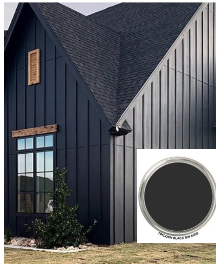
LP Smartside Board and Batten Siding and Trim, Painted SW Tricorn Black
