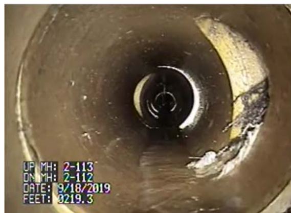
Figure 7 - Defective Tap: Roots
