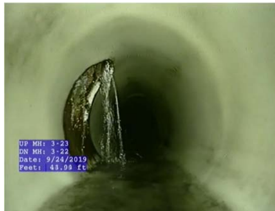
Figure 7 - Defective Tap: Roots
