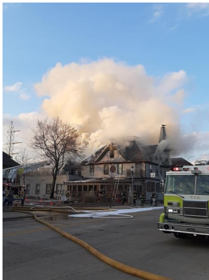
Fire Travels Through Void Spaces and into Attic
