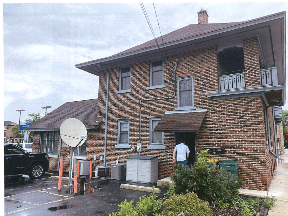
EXISTING BUILDING PHOTOS
