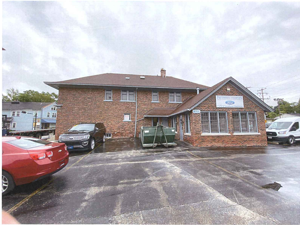
EXISTING BUILDING PHOTOS
