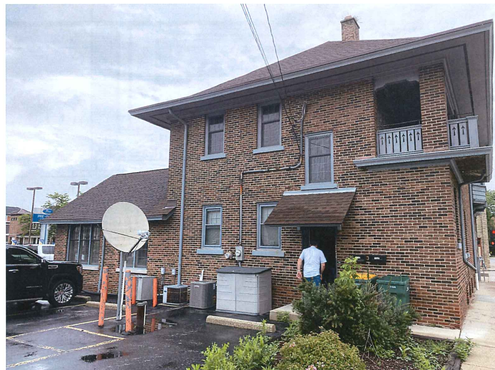
EXISTING BUILDING PHOTOS
