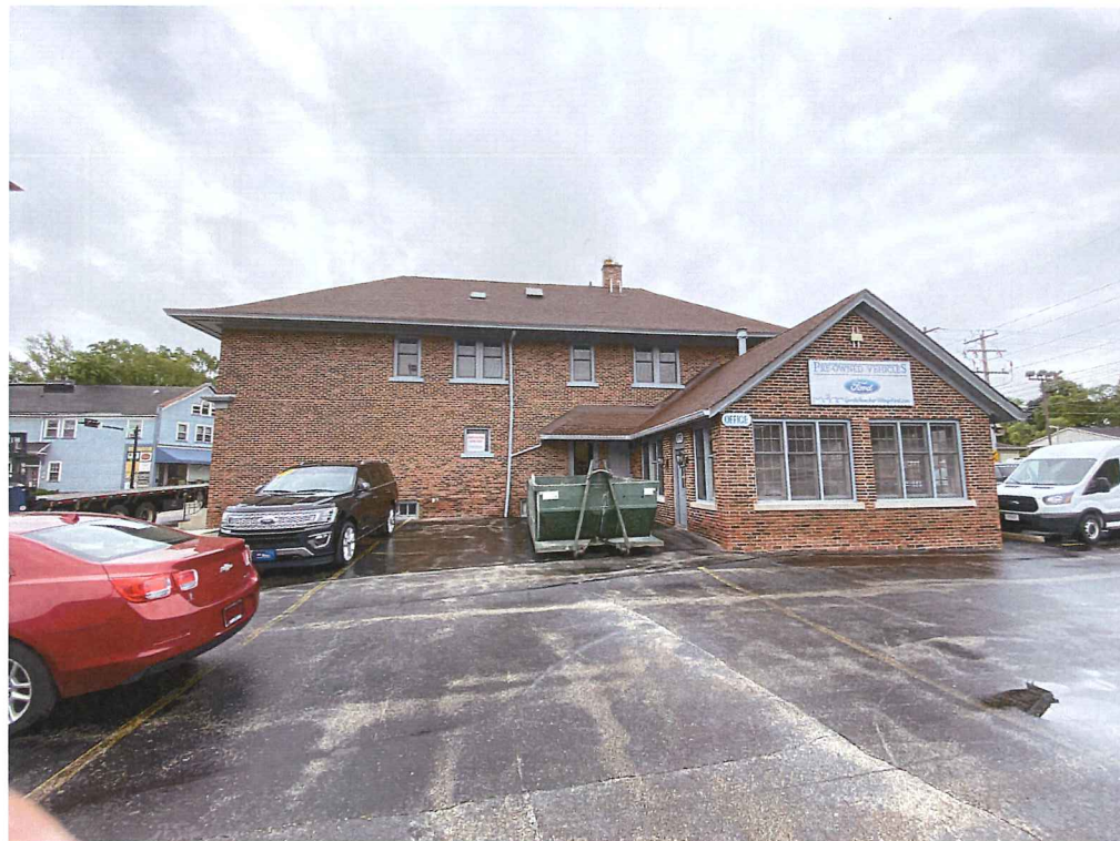
EXISTING BUILDING PHOTOS
