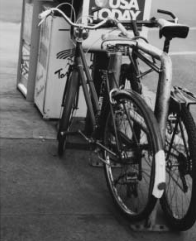
Inexpensive "hitching rail"-style bike racks work well for short-term parking for small numbers of bicycles. They should be installed in high-visibility locations.
